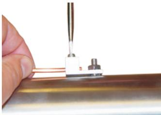
Ground/Bond the heater directly to the control box using the included #8 solid copper bonding wire.
