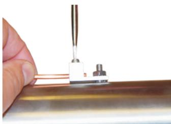
Ground/Bond the heater directly to the control box using the included #8 solid copper bonding wire.
