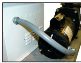
5) Route the other end of the conduit through and empty knock-out and secure with lock-nut. The cord inside will route up to the terminal strip inside the upper portion of the enclosure.
